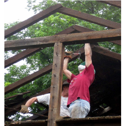
Harvesting roofing timbers from the farm house
